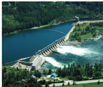
The Cora Linn Dam and FortisBC generating station on the Kootenay River; generating capacity is 49 MW. Source: FortisBC
